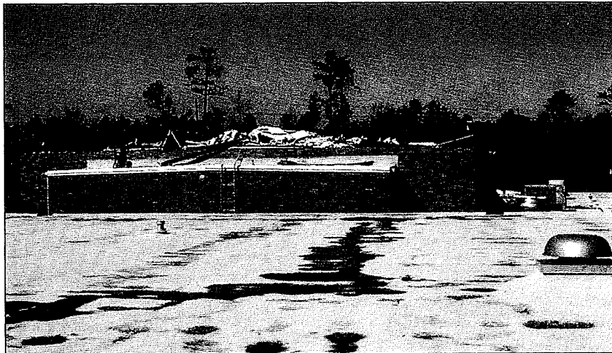
The spray polyurethane foam roof in the foreground on this high school in the Charleston area endured Hurricane Hugo, but the tectum deck of the gymnasium in the background gave way.
